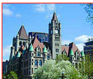
Landmark Center Located in downtown Saint Paul.
